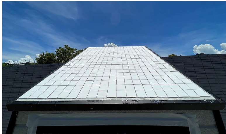
Application in a building envelope, with the white cooling ceramic applied on the roof. Credit: City University of Hong Kong
