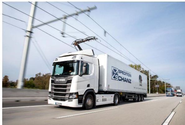
Siemens Mobility built an overhead contact line for electric trucks on a 6.2-mile stretch of Germany's autobahn.
